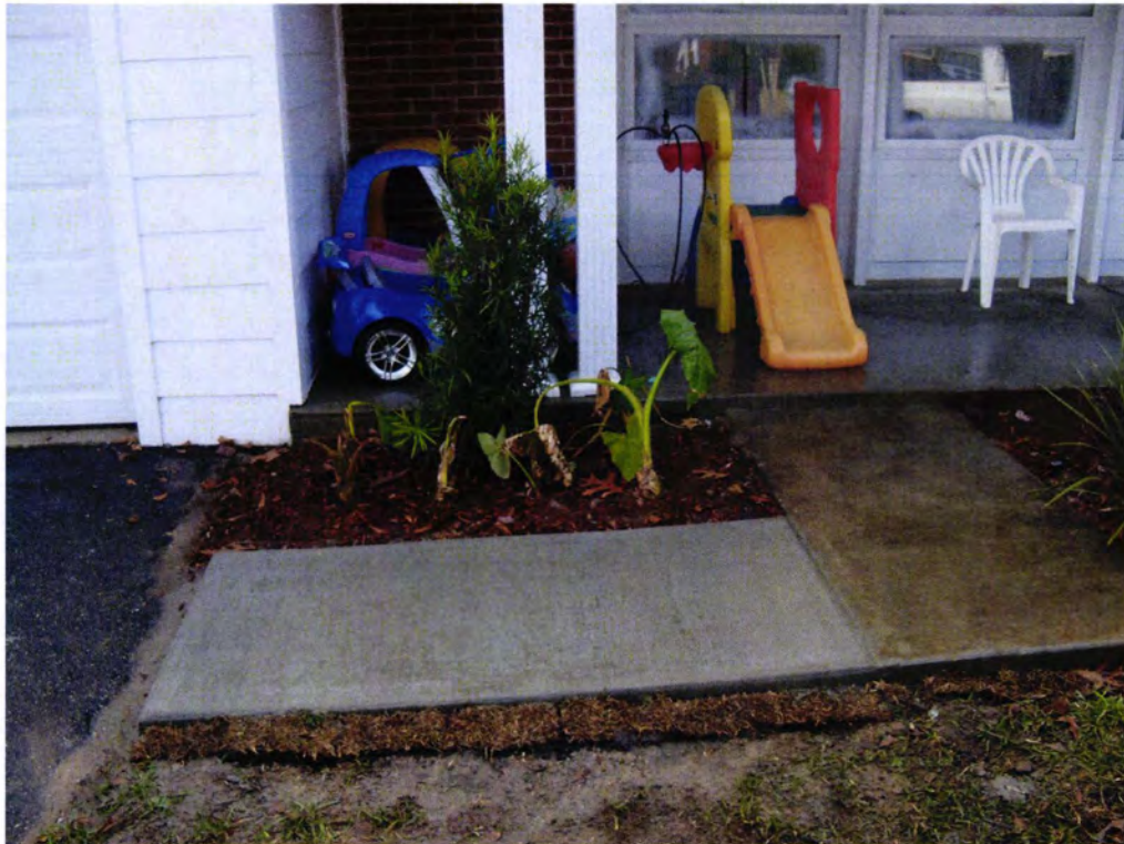
Picture 4: Site at completion of work.
